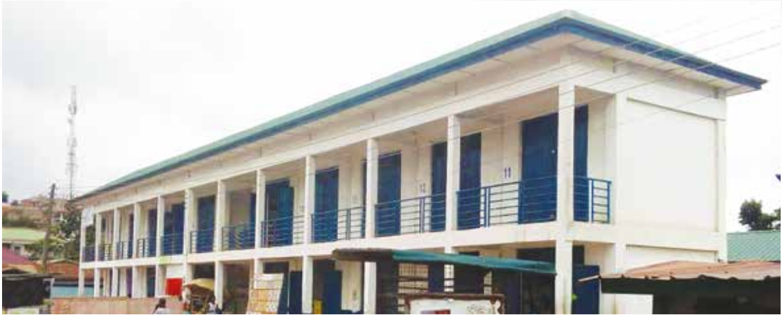
2-storey market at Yamoranza constructed by the SIF
